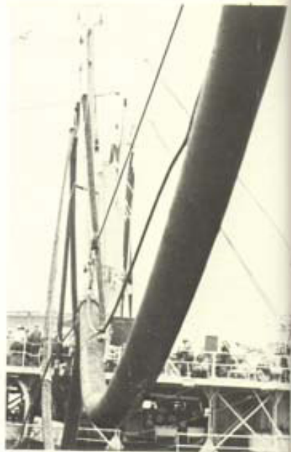
Like great anacondas, the fuel transfer hoses loop across the water from tanker to destroyer
