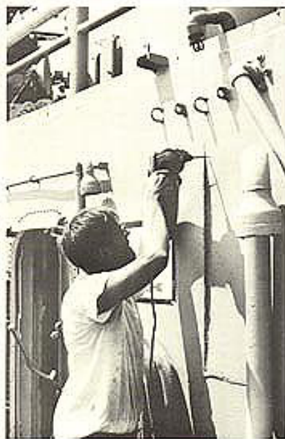
By checking equipment.....
